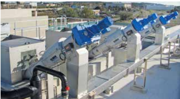
3 ROTAMAT® STAR units size 1000 with 1.5 mm perforation protecting the downstream membrane activated sludge plant.
