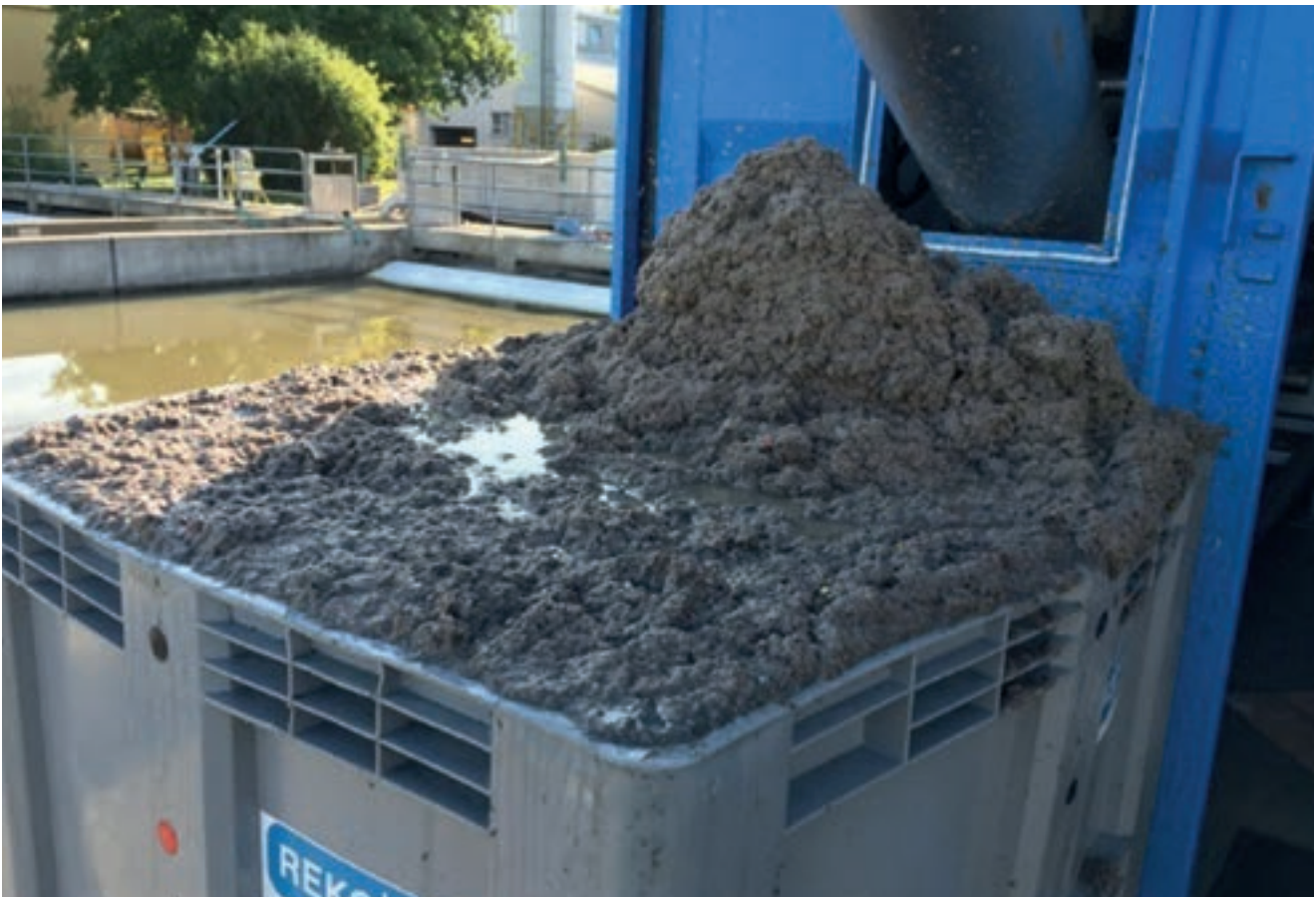
Screenings separated by the HUBER Drum Screen LIQUID mesh: The load to be handled in the biological treatment stage is reduced and more gas can be produced in the digester.
