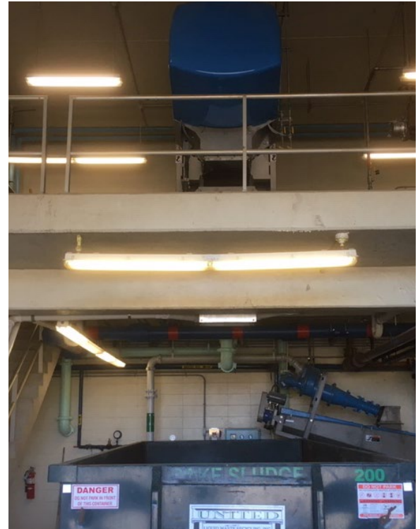
Q-PRESS® 620.2 configuration with cake outfall to disposal dumpster below.
