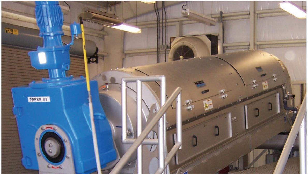
*"We looked at screwpress technology because it was new at that time and has distinct advantages over other technologies such as belt presses. The screwpress takes less energy, manpower and maintenance to operate so we went with it."*
