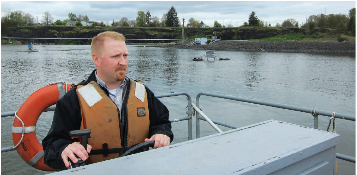
The Superintendent drives his boat by one of the SolarBee® mixers at the wastewater treatment plant.
