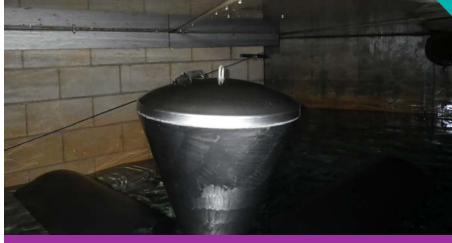
All SN Series are designed for operation in low headspace conditions.
