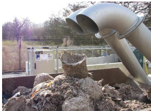
Fig. 7: Washed and compacted screenings
