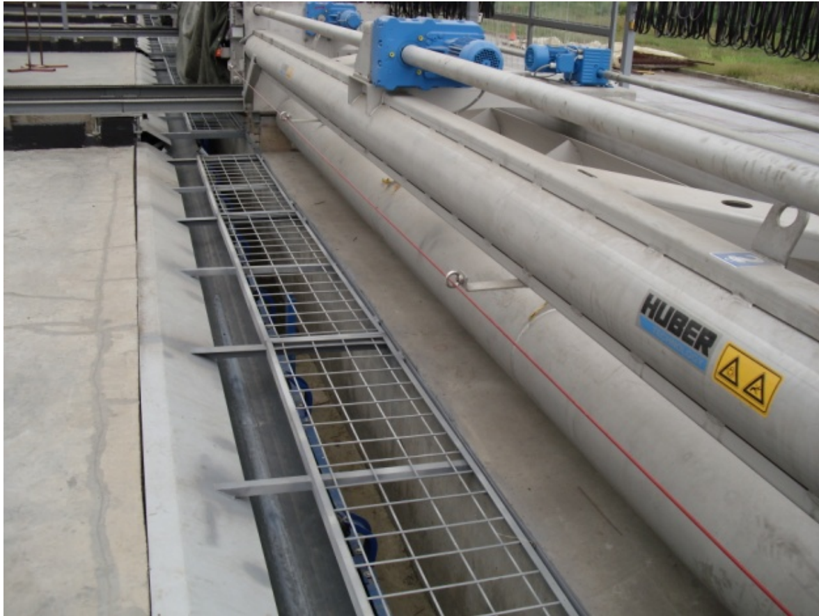
Figure 12: trench with discharge conveyor
