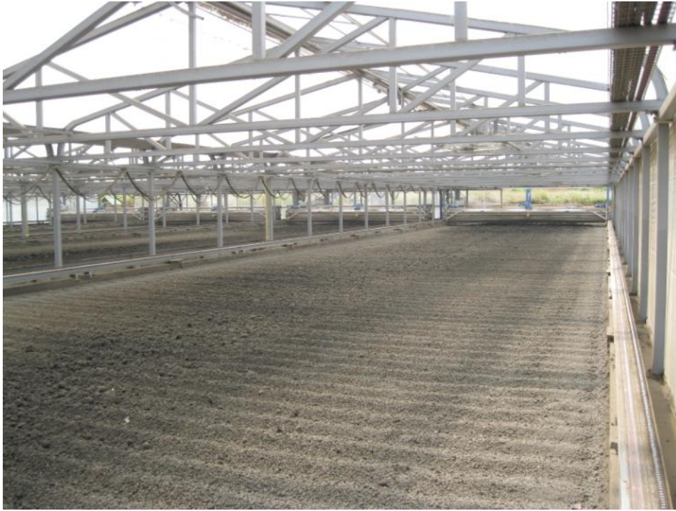
Figure 3: four dryer lines - SRT 9
