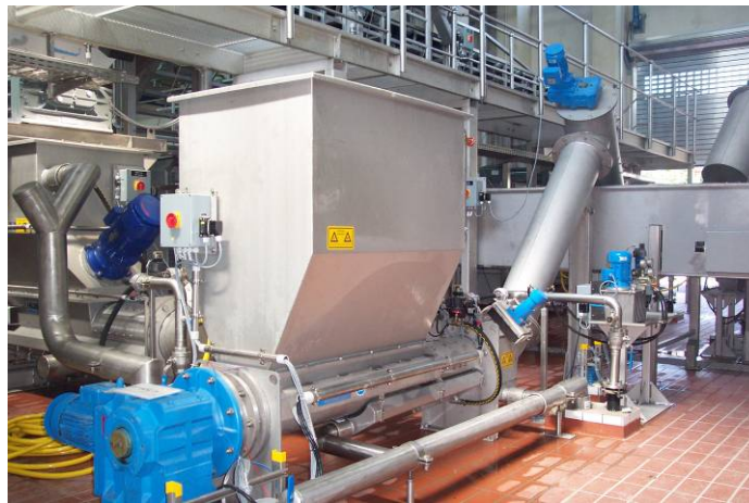
Figure 39 – Screenings washer/compactor with high pressure Compaction feature
