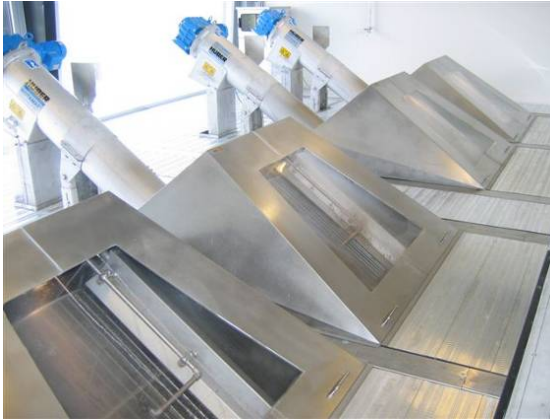
Figure 3- Ro2 installation in Denmark
