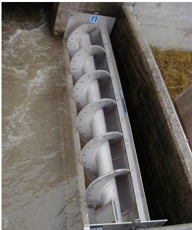
Figure 26 – Stormwater screen RoK1 installed at overflow weir
