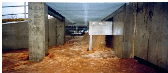
Figure 29 – Screen in operation during a heavy rain event
