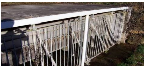
Figure 28 – Installation underneath a gutter
