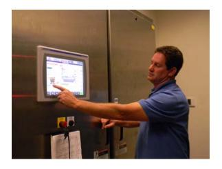
The technology enables Bill to work within his minimums and maximums to meet the needs or production goals of the plant. For example, Bill was asked to do what he could to help in reducing the plant's operational costs. Through tweaks in the drying process, Bill delivered savings in fuel use that wouldn't be possible without the transparency of Huber's BT Belt Dryer controls. Because of the precision of the dryer's dashboard technology, Bill literally sees the drying process as it unfolds and
