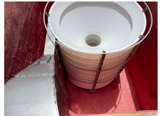
Fig. 7. Installed HeadCell® Stacked Tray Grit Separation System
