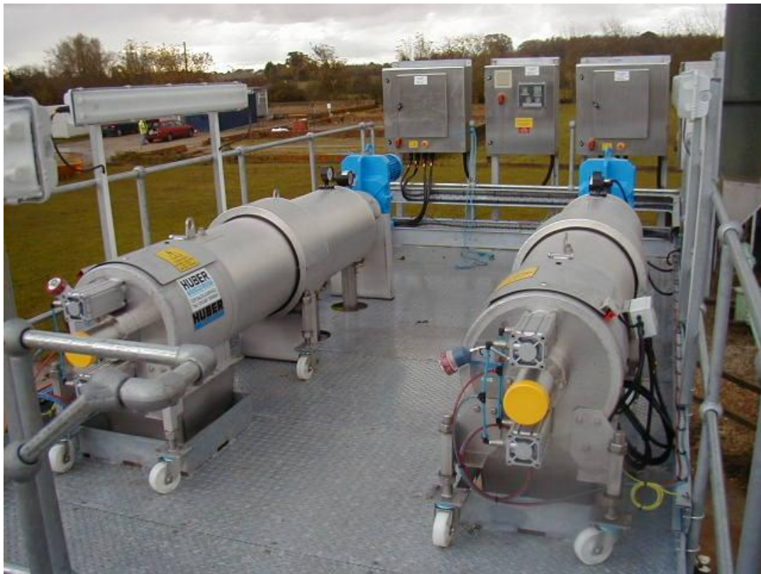
STRAINPRESS® installation, outdoor with frost protection
