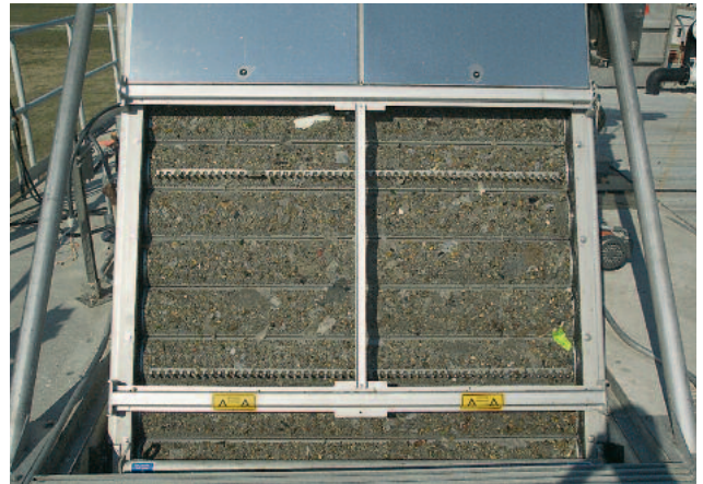
Screenings mat improving capture
