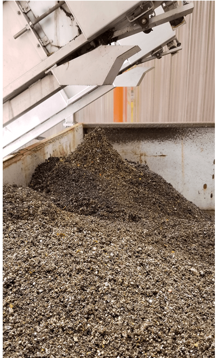
Airport WRF's Clean, Dry Grit Ready for Cost-Effective Disposal
