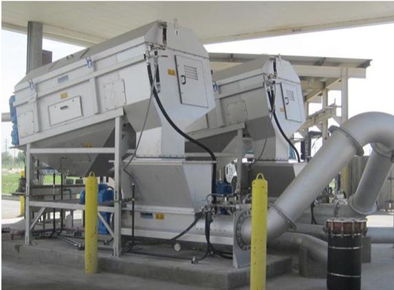
The “hybrid” implementation of Ro 3 and RoFAS units that SAWS now has works well to separate large solids and grit from the septage that passes through the station. There are back-ups units for both the Ro 3 and RoFAS on stand-by so that SAWS is always online.
