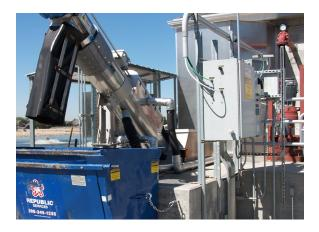
"We need to make the flow entering the membrane bioreactor as clean as possible. Keeping the Muffin Monster didn't make sense – even if it was repaired to its performance potential." -Ken Vose, Plant Operator
