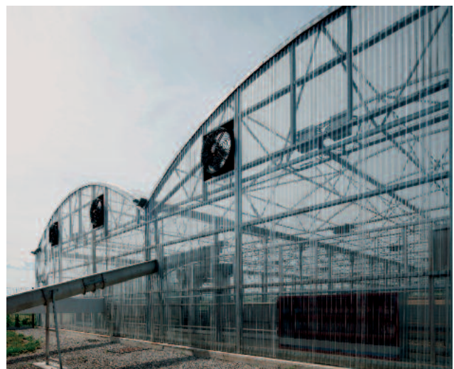
Automated sludge feeding with a screw conveyor
