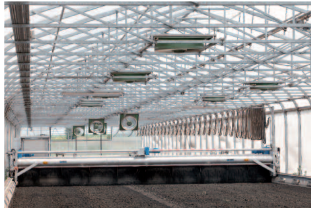
The sludge turner on its way through the greenhouse
