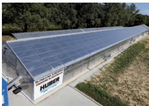
Greenhouse with ridge flap for climate control
