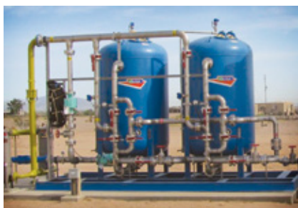
Pictured: Use of E33 media in typical Adsorption Package Units (APU) and in Modular System installations.
