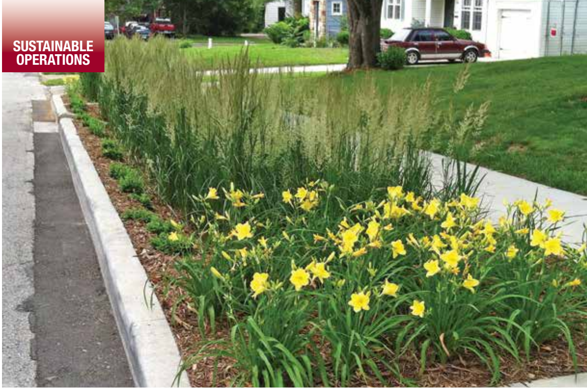
KC Water uses green infrastructure, including rain gardens planted in the parkways between the sidewalk and street, to help attenuate stormwater flows.
