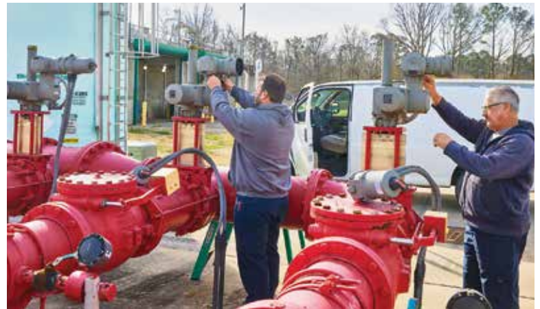
Joe Barnett (left) and Bob Martin perform maintenance on AUMA actuators.
