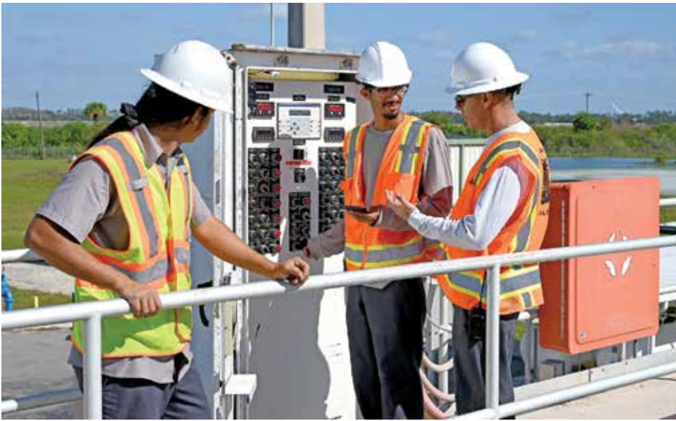
From left, operators in training Michael Rogers and Jose Gonzalez, and operator Israel Guadarrama backwash the filters.
