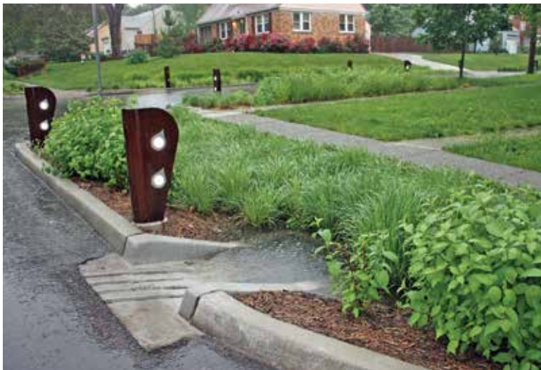
Green infrastructure projects help KC Water capture a higher percentage of wet-weather flows before the water overwhelms the collection system.
