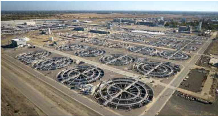
The secondary sedimentation tanks at the Sacramento Regional County Sanitation District wastewater treatment facility
