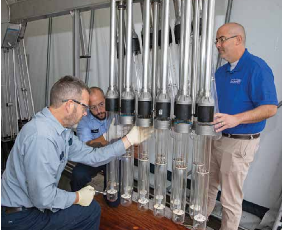
From left, Tom Bjorkland, Mike Wood and LeMay remove hydraulic wipers from UV light bulbs as the disinfection system (TrojanUV) is taken offline for the season.
