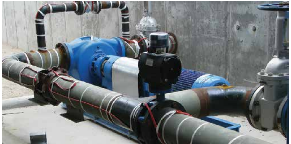
PHOTOS COURTESY OF EMERSON
