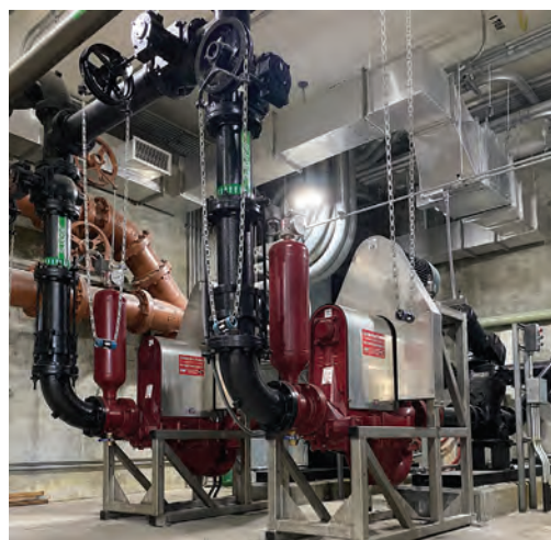
ABOVE: Two centrifuges (GEA Group) dewater biosolids delivered by newly installed Double Disc Pumps from Penn Valley Pump. LEFT: The Double Disc Pumps are designed for ease of maintenance with maintain-in-place hinged housings that enable quick disassembly and reassembly.
