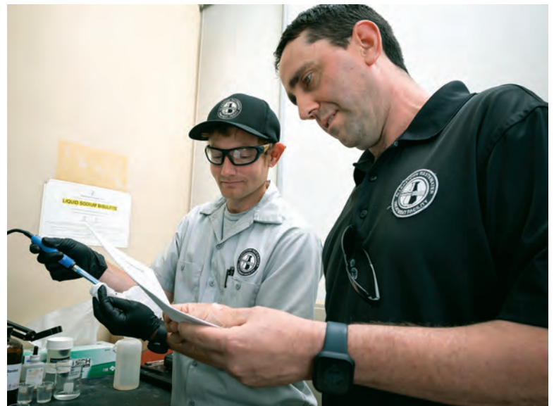
Hobie Shireling, operations and maintenance technician, and Backman perform calibration and maintenance on the pH monitoring system in the dechlorination room.
