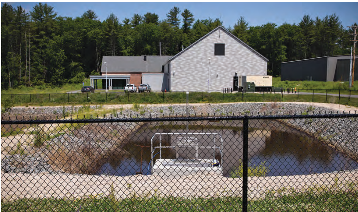
The main operations building at the Durham Water Treatment Plant, which also serves the University of New Hampshire.
