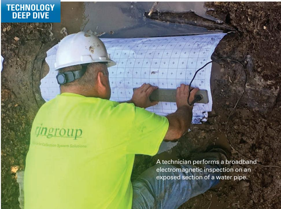
A technician performs a broadband electromagnetic inspection on an exposed section of a water pipe.
