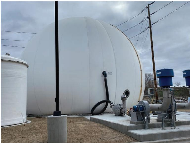
This “bubble” tank stores biogas at the plant.
