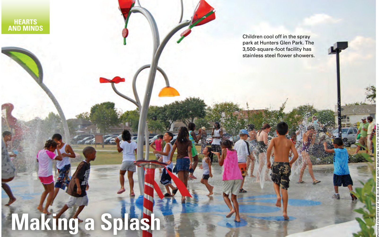
PHOTOS COURTESY OF THE BLUE RIDGE WEST MUNICIPAL UTILITY DISTRICT
