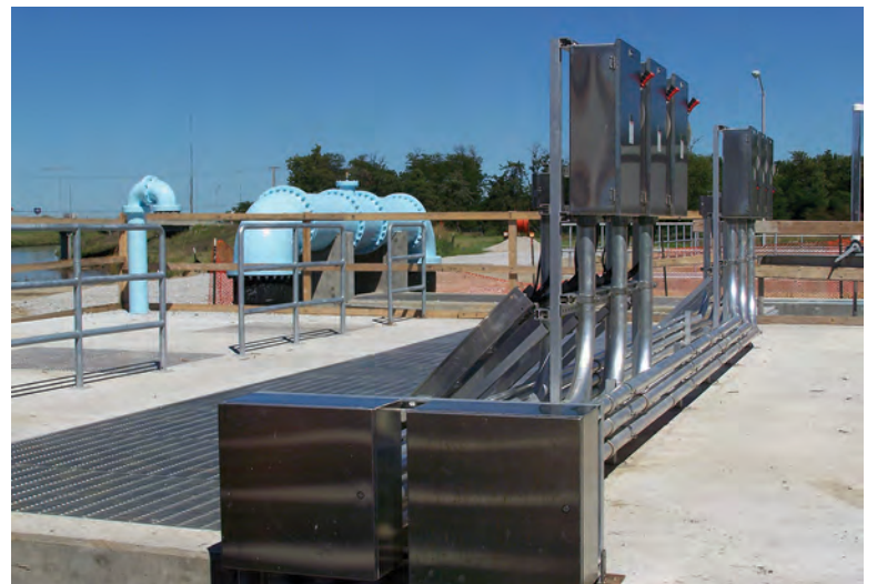
Six pumps (Flygt) at the submersible pump station automatically divert effluent to the Centralized Renewable Energy System on the Innovation Campus through a 30-inch ductile iron pipe. The effluent is returned to the plant for discharge to Salt Creek.
