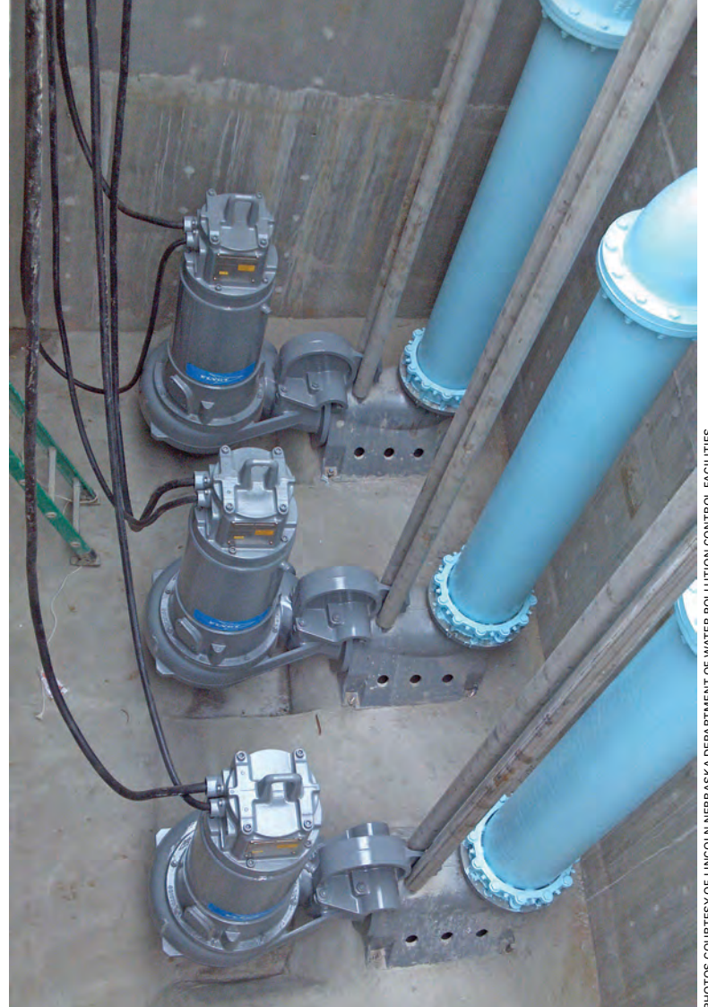
Six pumps (Flygt) at the submersible pump station automatically divert effluent to the Centralized Renewable Energy System on the Innovation Campus through a 30-inch ductile iron pipe. The effluent is returned to the plant for discharge to Salt Creek.
