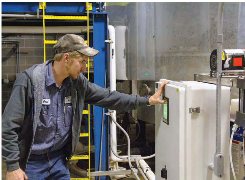
Josh Peaster adjusts the settings of a polymer makedown skid. GreenWhey Energy uses polymer in its two dissolved air flotation (DAF) units.
