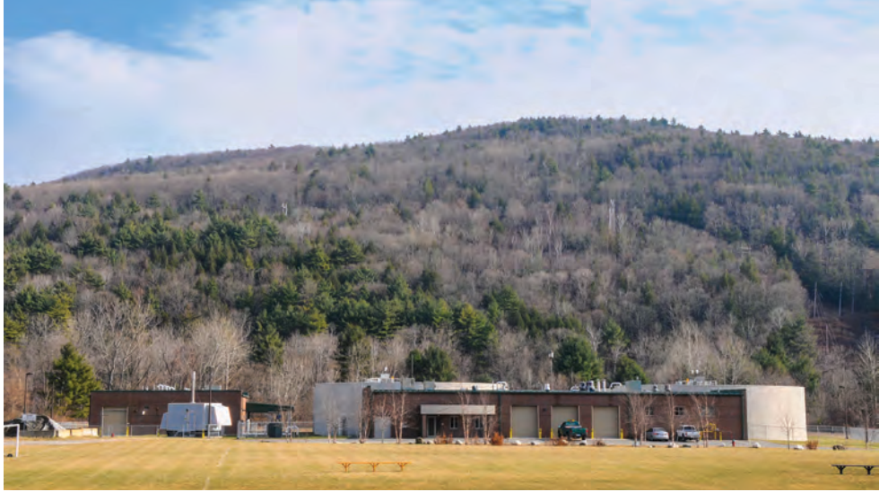
The Lee Wastewater Treatment Plant is located in the picturesque Berkshire Mountains of western Massachusetts. (Photography by Ed Collier)
