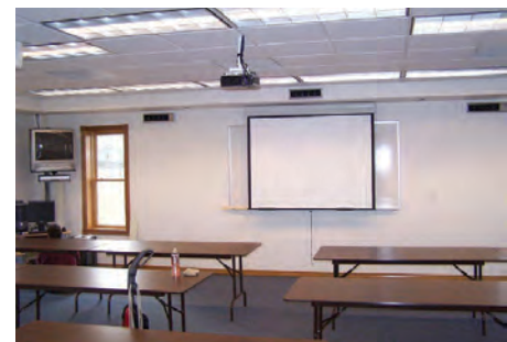
A refurbished conference room is among the amenities of the upgraded facilities.
