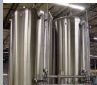
High Solids Anaerobic Digestion (HiSAD) System from Infilco Degremont
