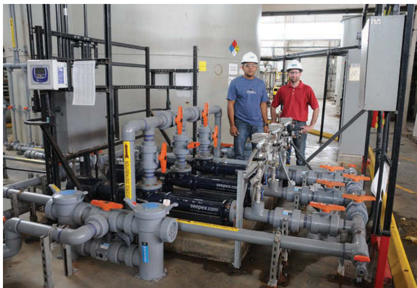
Zainool Ali, left, plant superintendent, and Bill Sedutto, process engineer, in the glycerol storage and pumping room. A $2 million research and development program prevented a $30 million expenditure to reduce nitrogen discharges into Jamaica Bay.
