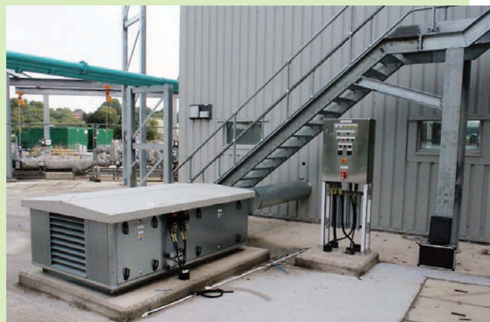
Terminodour odor control system from CSO Technik (distributed by Kusters Water)
