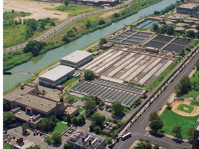
The 85 mgd 26th Ward treatment plant in New York City is the first site in the nation to use glycerol to reduce nitrogen in effluent to protect the sensitive Jamaica Bay estuary.
