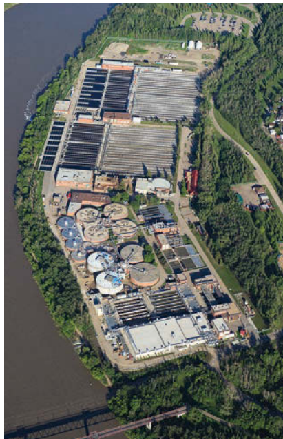
The 82 mgd Gold Bar Wastewater Treatment Plant in Edmonton operates an ultrafiltration membrane treatment process as part of a treatment train that supplies reclaimed water to an oil refinery.
