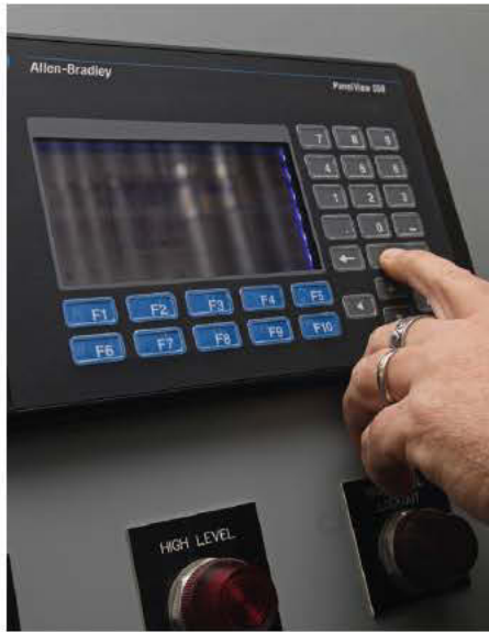
BELOW: The control panel (Allen-Bradley/Rockwell Automation) for the vacuum sewer system. RIGHT: Operator Chris McKernan tests samples in the lab using a Hach DR 2800 portable spectrophotometer.
