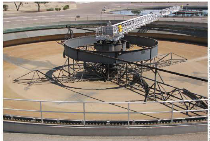
Optimization of the clarifiers, including the addition of Stamford baffles (NEFCO) has helped reduce BOD load before the aeration phase and so reduce the use of blowers.
