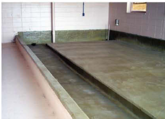
LEFT: The sludge transfer room during preliminary cleaning and preparation. RIGHT: The rehabilitated and protected substrate surface after application of SprayWall.
