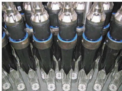
FIGURE 2. Vortex mixers mounted on quartz sleeves housing medium-pressure UV lamps provide additional mixing and direct the low-UV-transmittance water toward the high-intensity light source.
