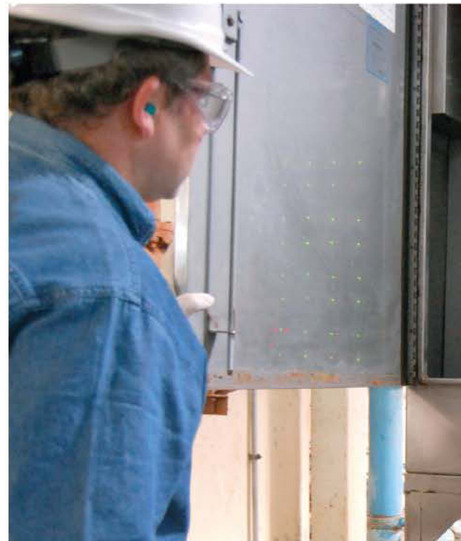
Operations and maintenance technician Mark Byrns prepares to clean UV light panels, part of the Newtown facility's Fisher & Porter disinfection equipment (Ironbrook Partners). (Photography by Margaret Waage)
