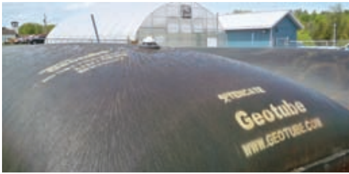
Filtrate from the dewatering process pours off a Geotube container.
