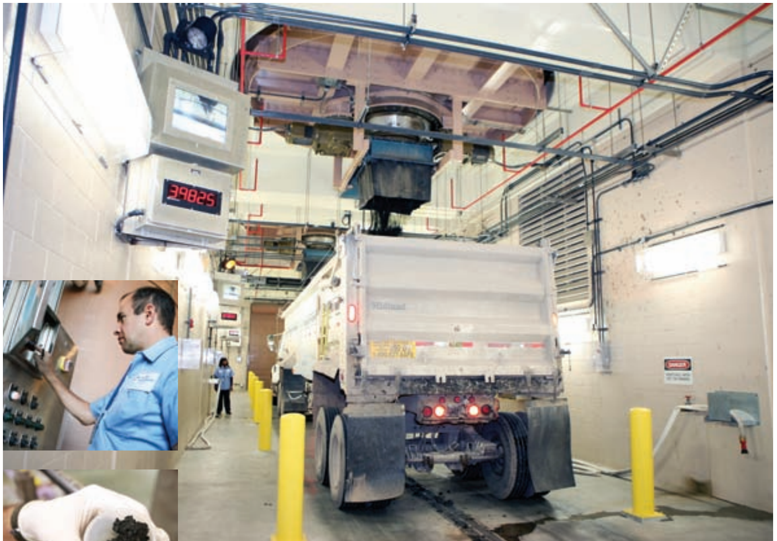
ABOVE: A Republic Services truck is filled with dewatered solids. UPPER INSET: Kevin Forgione, operations technician 2. LOWER INSET: A sample of dewatered cake.
