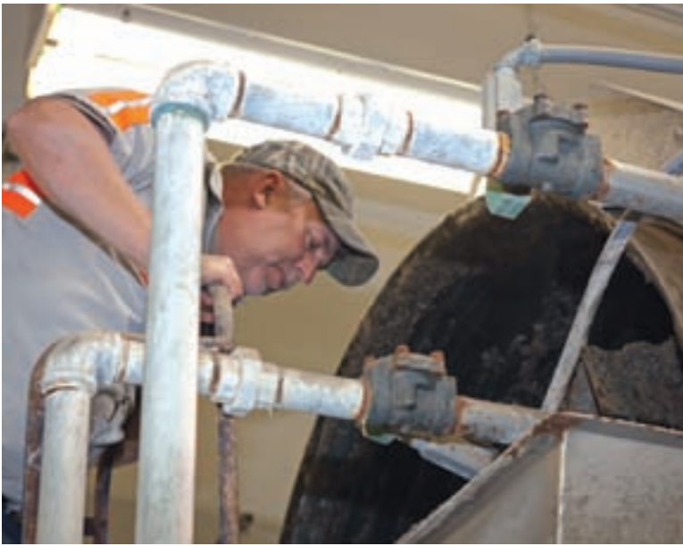
Kevin Massmann, operator 3, inspects the drum screen in the influent headworks.
