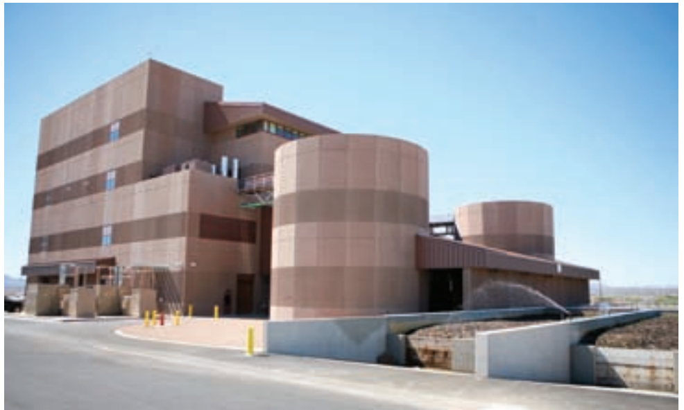
The biosolids dewatering building at the Clark County Water Reclamation District. (Photography by Ronda Churchill)
