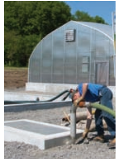
George Griffith of George's Septic Pumping in Eganville discharges digested sludge to the 10,000-gallon subsurface holding tank.
