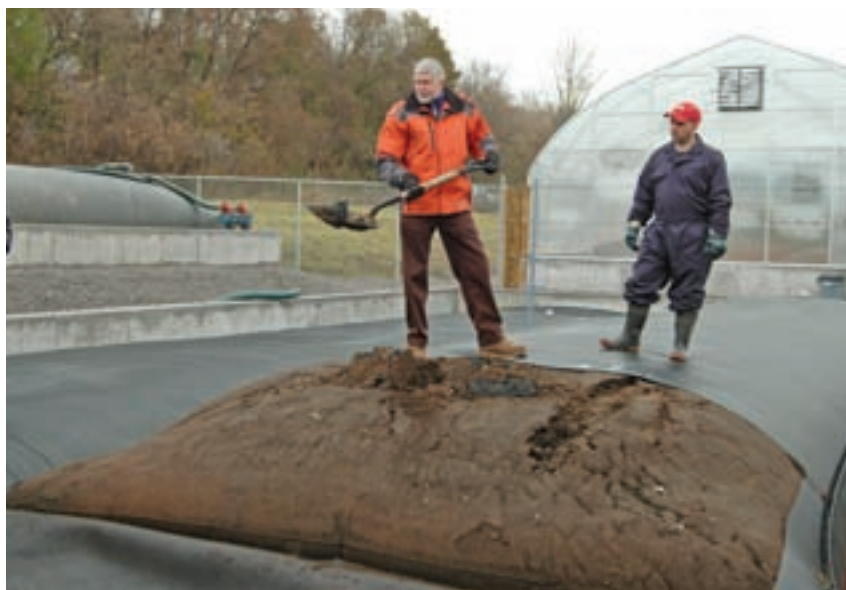
Andrew Polley, left, environmental project manager, and Dave Loader, Eganville Sewage Treatment Plant operator, evaluate the dewatered material from a TenCate Geosynthetics Geotube container.
