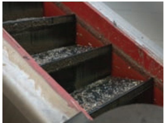
The Eutek Grit Snail dewatering escalator supplied by Hydro International, showing the cleated belts that carry and dry grit removed from the wastewater.
