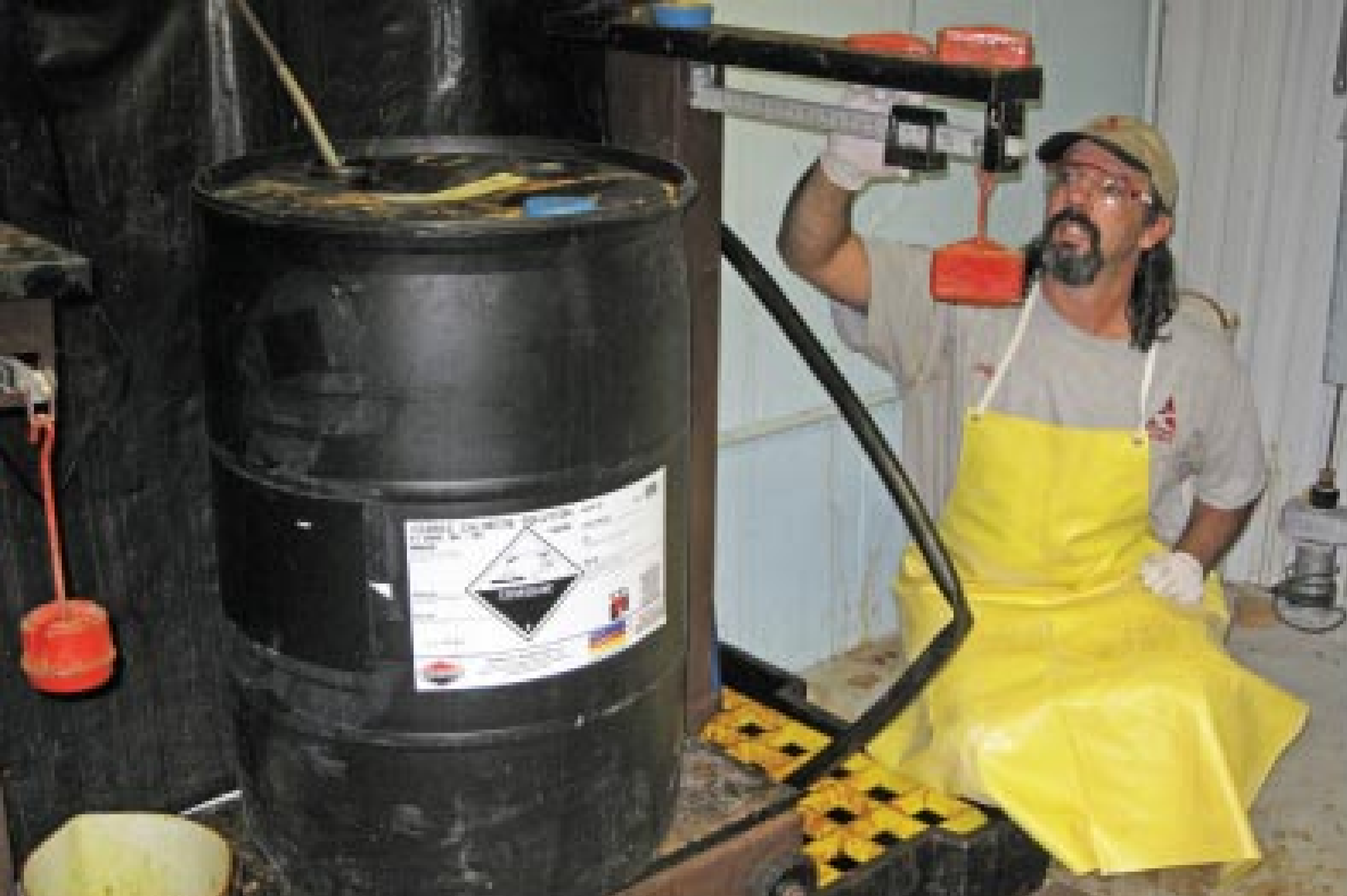
With the addition of sodium hydroxide at an automatically controlled rate, the facility consistently achieves pH 7.0 in final effluent.
