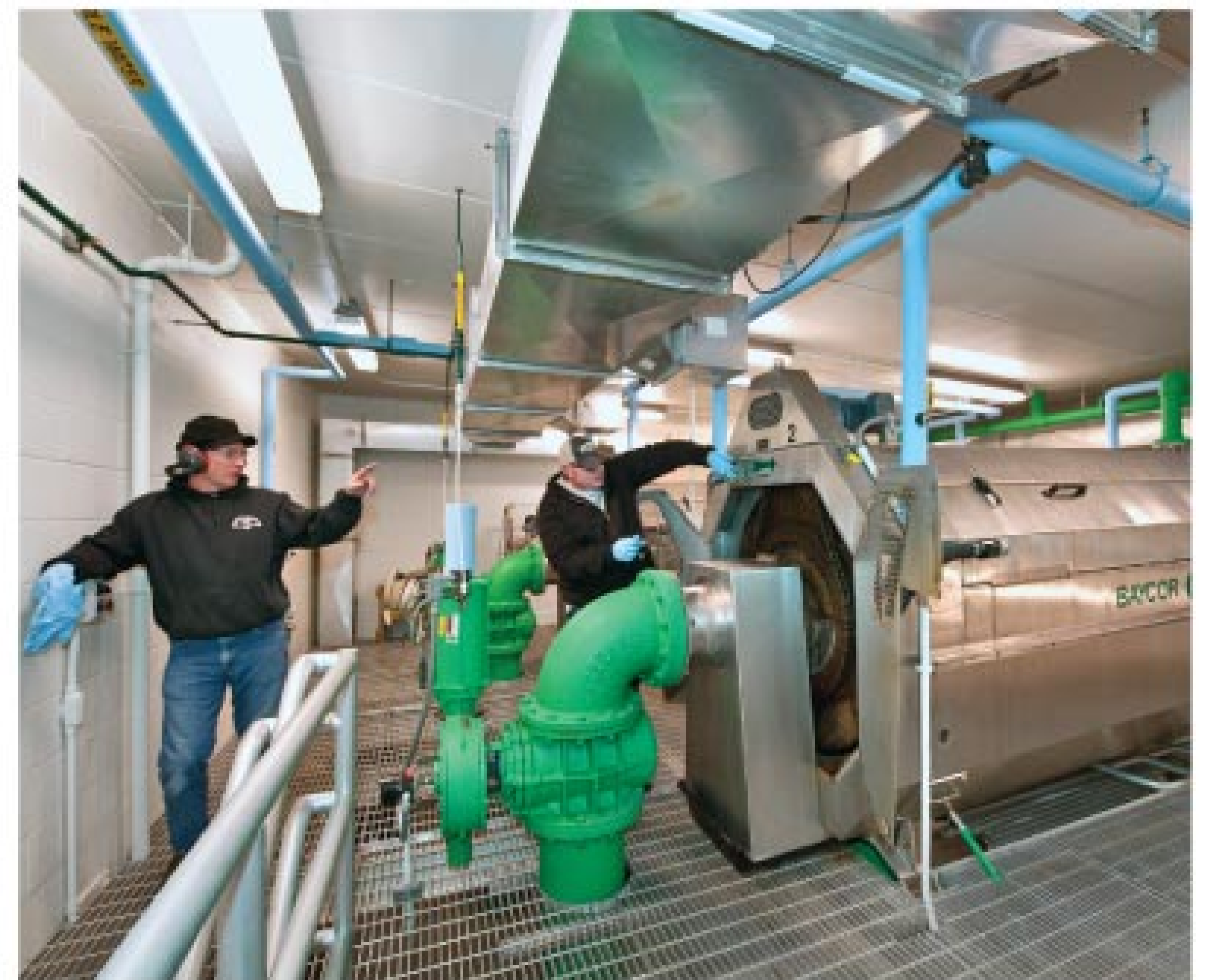
North Liberty plant operator II Tom Arey and plant operator I Drew Lammers perform routine maintenance on one of the Baycor screens in the MBR facility.
