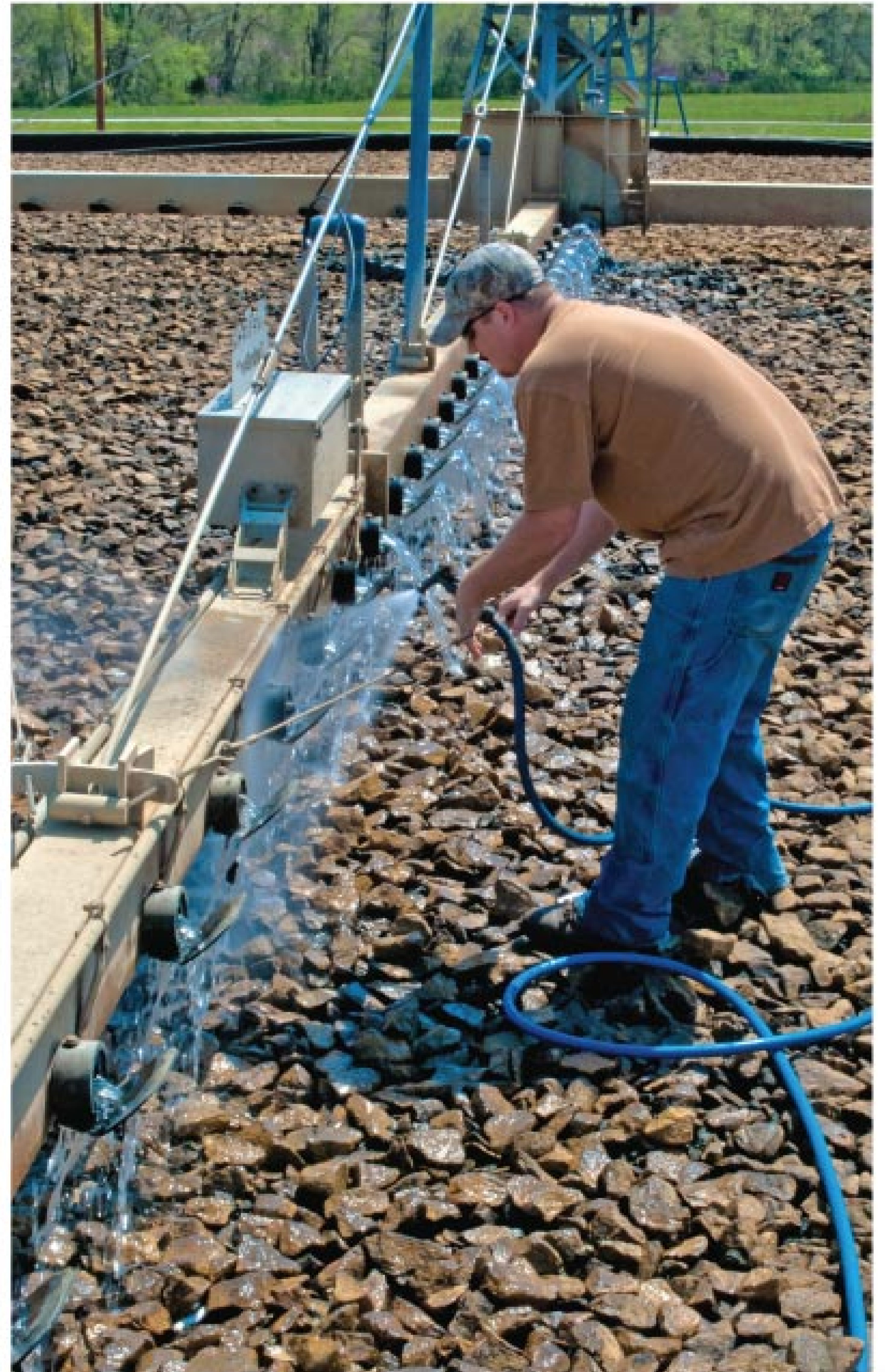
LEFT PHOTO: Superintendent Mike Brown checks the plant's UV disinfection system from Aquionics. LOWER PHOTO: Grant Gilmore cleans the outputs on a four-arm drip distributor from WesTech Engineering Inc.
