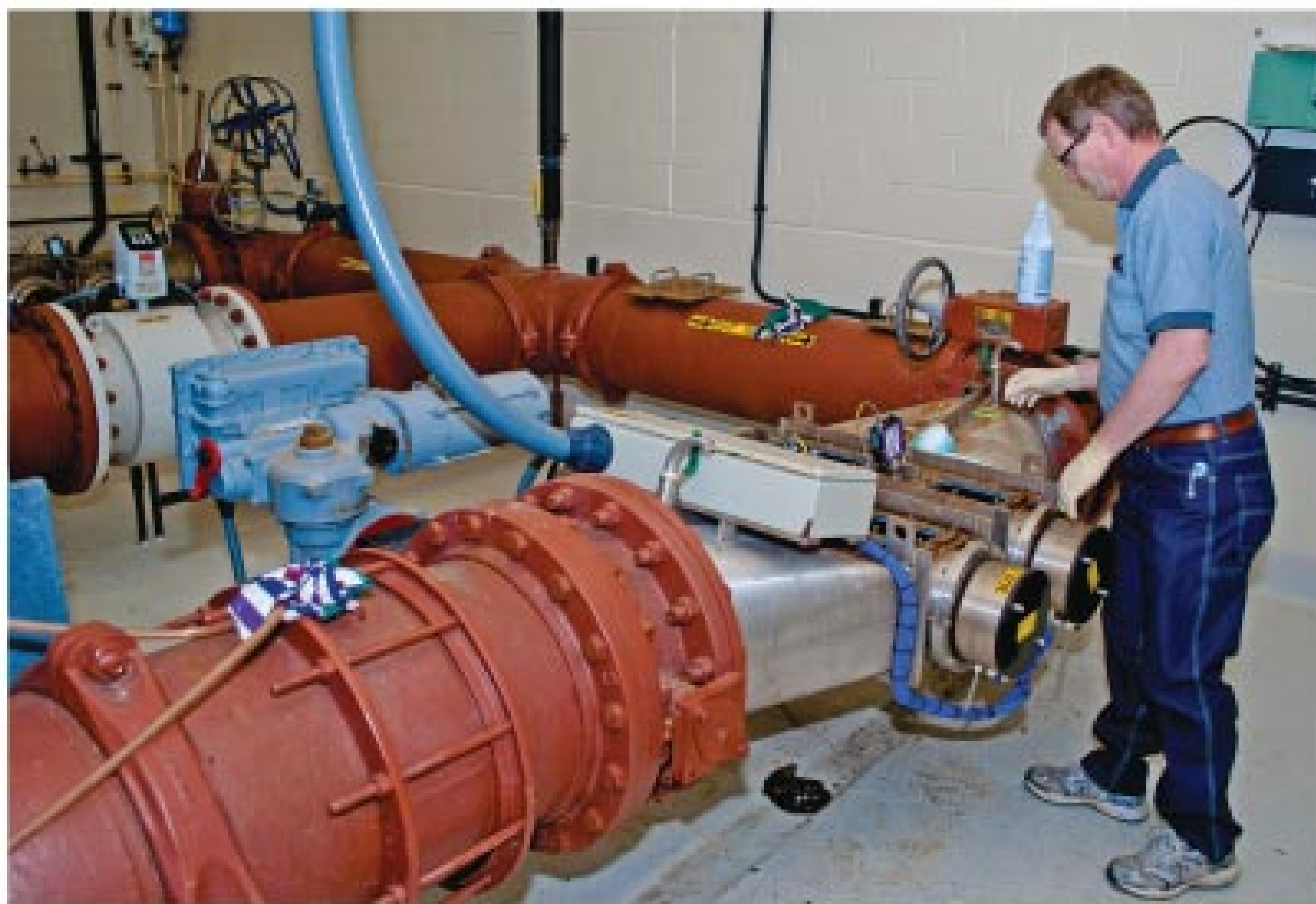
LEFT PHOTO: Superintendent Mike Brown checks the plant's UV disinfection system from Aquionics. LOWER PHOTO: Grant Gilmore cleans the outputs on a four-arm drip distributor from WesTech Engineering Inc.
