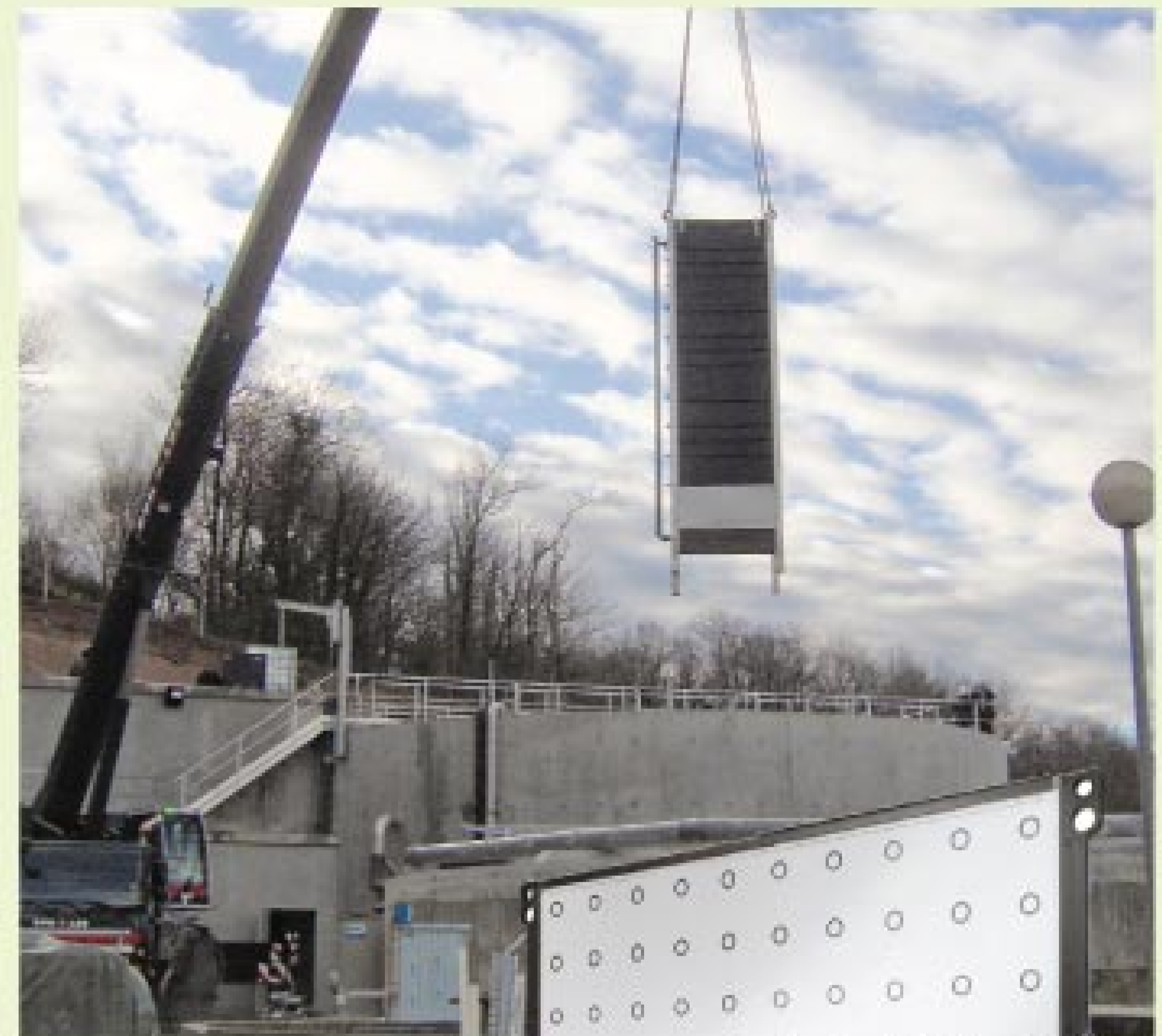
ClearLogic membrane bioreactor filtration system from WesTech Engineering
