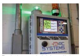
The plant instrumentation includes a multipoint alarm system (RC Systems).
