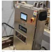
Plant effluent undergoes UV disinfection (Glasco UV)
