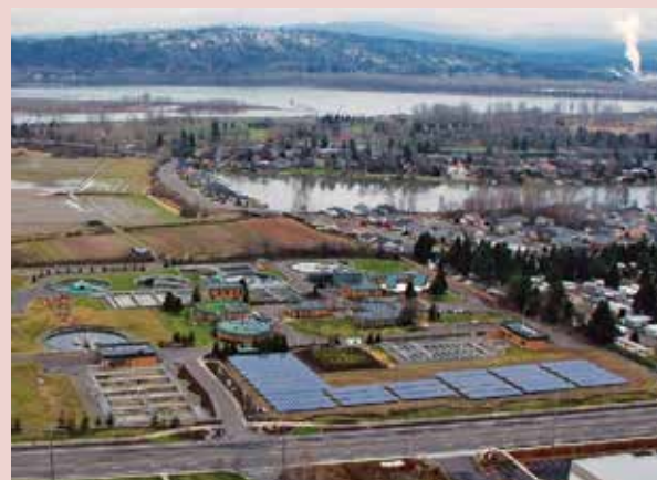
An aerial view of the Gresham treatment plant shows the 475 kW solar power array that helps the facility achieve net-zero energy.
