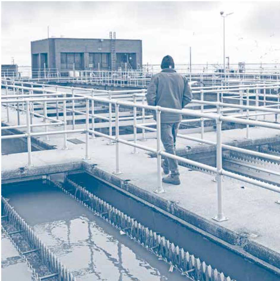
The Bergen Point Wastewater Treatment Plant uses an activated sludge process with 40 mgd design capacity and plans to expand to 50 mgd.
