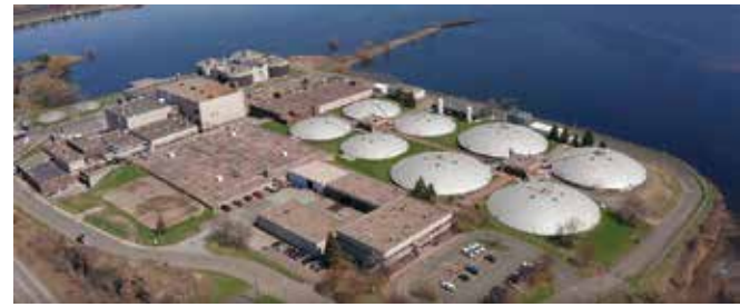
Aerial view of the Western Lake Superior Sanitary District wastewater treatment plant. The effluent flows along the pier into the St. Louis River.
