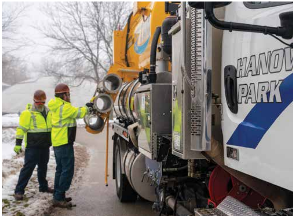
Brian Wurst and Scot Lichtenberger with the city's Vactor combination sewer cleaning truck.
