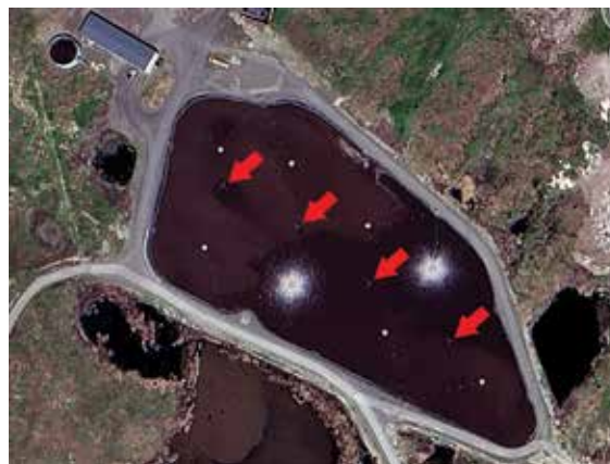
An aerial image shows location of the four new mixers as well as the eight aerators. After the mixers were installed to take over the mixing function, only two of the eight aerators operate at a time.
