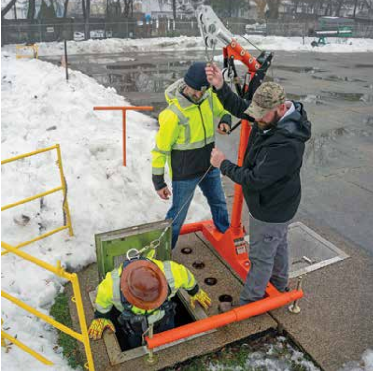
Chris Rebone, in black, and operator Lance Winterland use confined-space entry equipment in lowering Mike Klaus into a treatment plant storage tank for an inspection.
