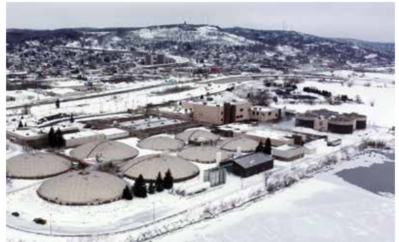
Warm effluent from the plant creates an area of open water in the frozen St. Louis River in Duluth. The city is using a U.S. Department of Energy grant to study the feasibility of using heat from the effluent to heat buildings in a commercial district.
