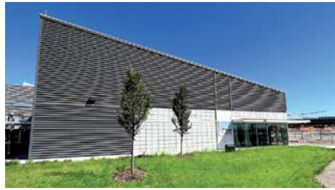
The National Western Center built this central utility plant next to a buried sewer line. Heat exchangers inside transfer heat from wastewater to a closed loop that supplies heated water to several buildings.
