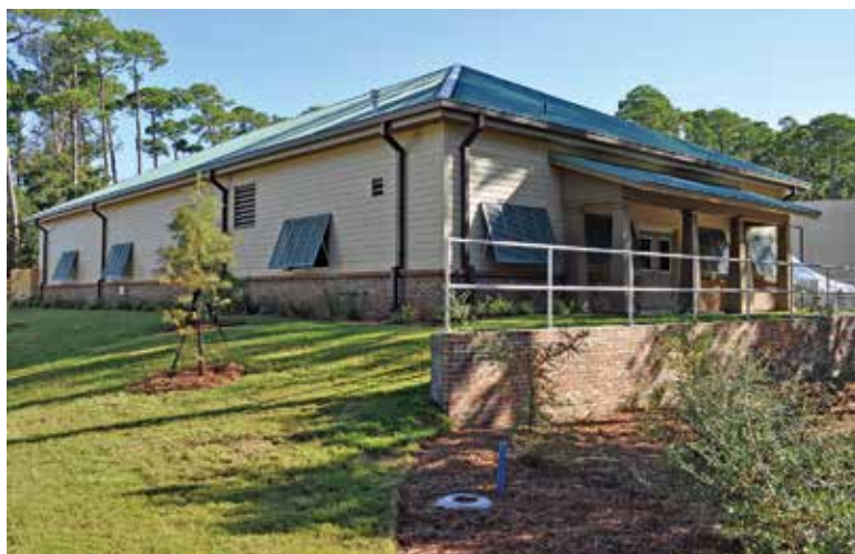
The certified LEED Silver water treatment building on Dauphin Island is landscaped to minimize stormwater effects and the need for irrigation.
