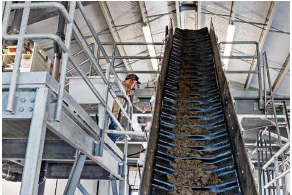
Sludges from the Central Davis district treatment process are converted to biosolids for land application and compost.
