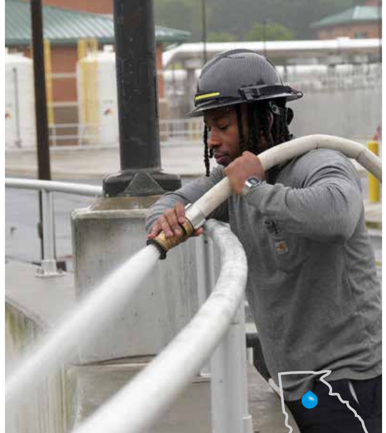
Edward Appiah cleans the weirs of a secondary clarifier.
