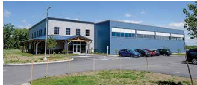
The Saco River Drinking Water Resource Center replaced a water treatment plant built in 1884.
