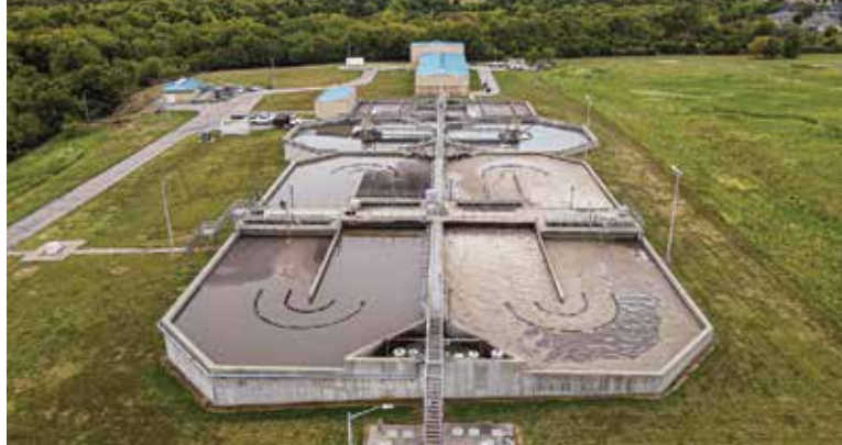
The Kill Creek treatment plant (2.5 mgd design) uses a Bio-Denitro phased oxidation ditch secondary process (Veolia Water Technologies).
