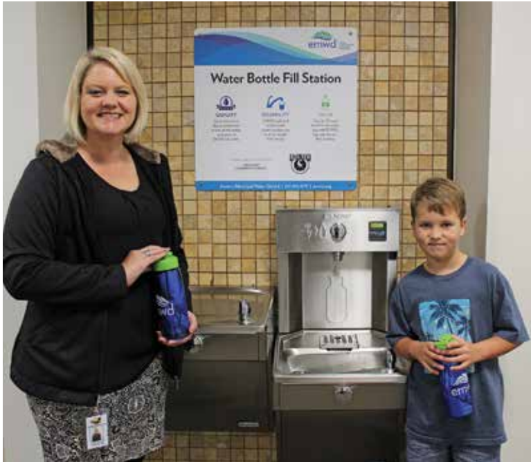
Students and staff at schools can stay hydrated with cold tap water from newly installed water bottle filling stations like this one provided by Eastern Municipal Water District. The stations help reduce usage of plastic throwaway water bottles.
