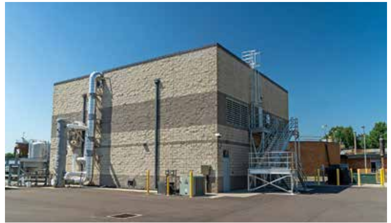
The new cogeneration facility at Willow Lake Wastewater Pollution Control Facility, Salem, Oregon.
