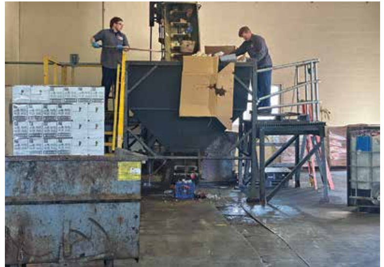
Hermitage Water Pollution Control Plant workers load packaged food into the Scott Equipment Turbo Separator.
