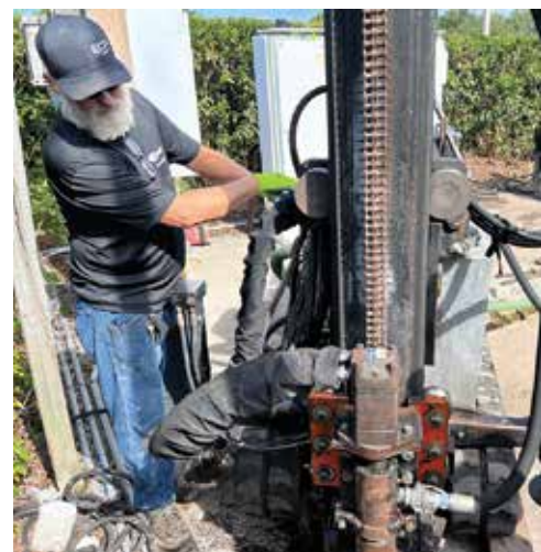
A special DHIG rig is used in part to advance the injection casing to the desired depth.
