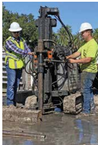
Deep horizons general grouting is a method of chemical grouting that enables injection at depths far exceeding previous limits.
