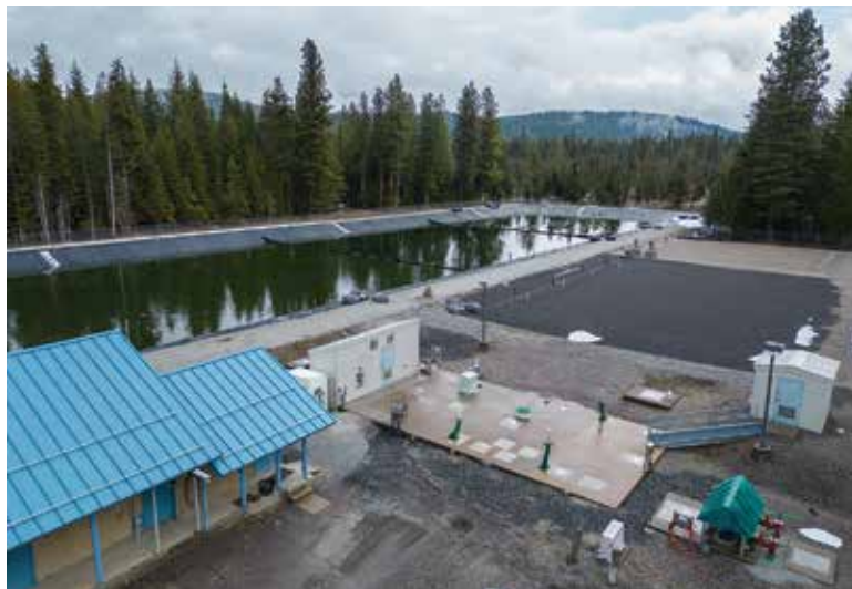
The Lake Wenatchee Wastewater Treatment Plant received effluent pumped in from some 240 individual septic tanks.
