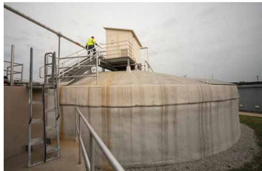
Royce's daily tasks include inspections of plant equipment and infrastructure.
