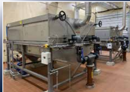
Dual 4 x 10 Rotary Drum Thickeners
