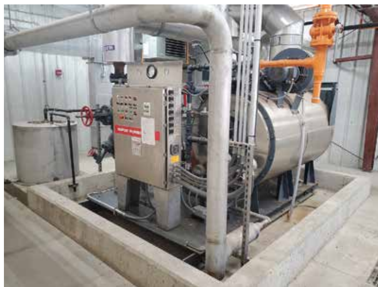
The Vapor Power thermal oil heater for drying biosolids is fueled by biogas, supplemented by natural gas when needed.
