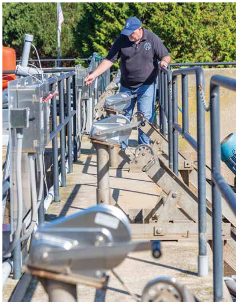
Scott Goodinson operates the oxidation ditch blower via hand-off-auto (HOA) switch. Blowers and mixers are from Aeration Industries (Newterra); Square D control boxes (Schneider Electric) govern the HOA and safety disconnect switches.
