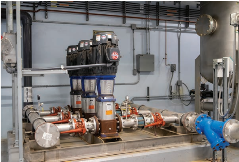
Finished water pumps (top photo) and air/water saturation pumps (lower photo), both from Goulds Water Technology, with motors from US Motors (Nidec).
