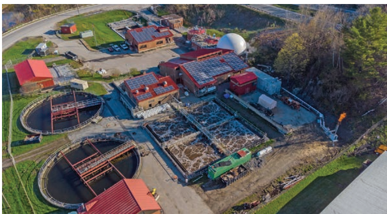
The biogas goes directly to dual-fuel boilers. The Montpelier plant produces more biogas than it can use in summer. The excess is flared (lower right of the photo), but the staff is developing a project to use more of the gas.
