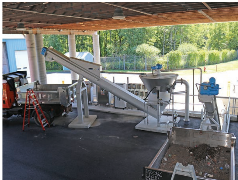
The catch basin sand cleaning process includes a grit dosing screw and hopper, wash drum and conveyor, all supplied by HUBER Technology.
