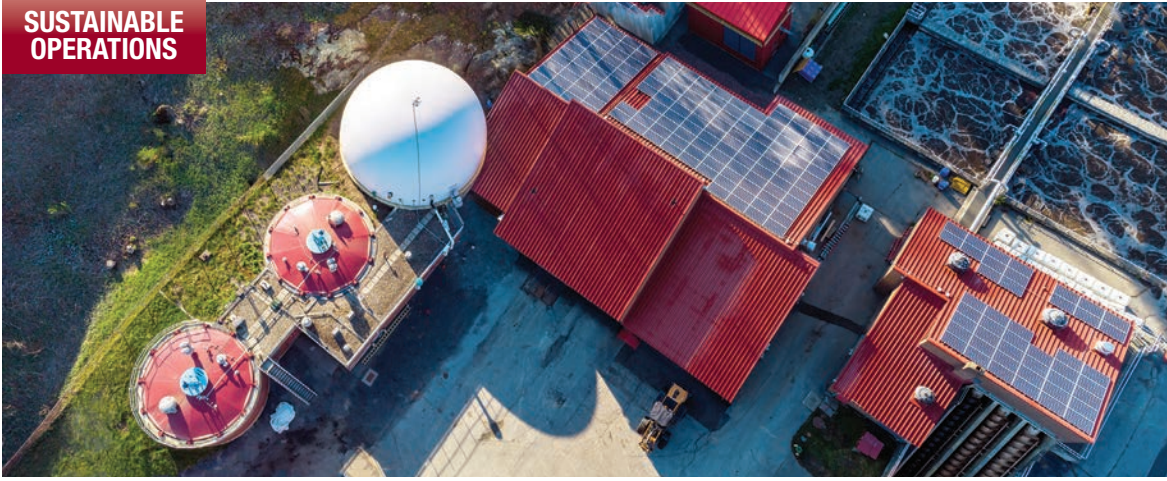
Three digesters at the Montpelier Water Resource Recovery Facility were fitted with new covers, two with Ovivo linear motion mixers, and the third with an Ovivo dual-membrane cover to store biogas produced from high-strength organics.
