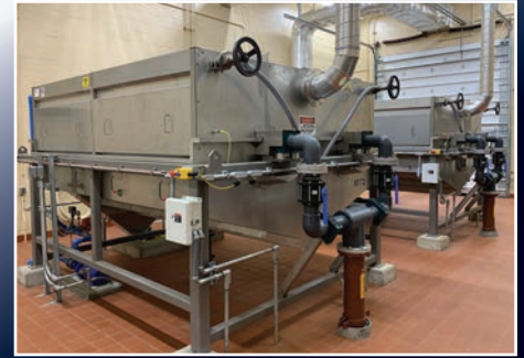
Dual 4 x 10 Rotary Drum Thickener
