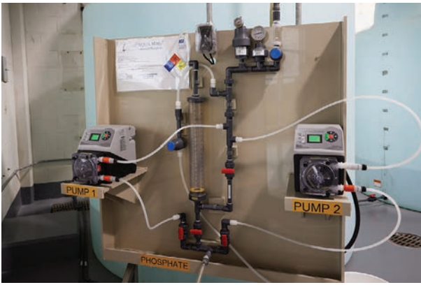
Peristaltic chemical metering pump for liquid phosphate was supplied by Blue-White industries.
