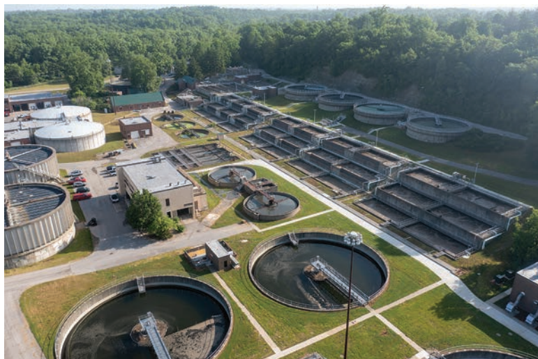
The Richmond Wastewater Treatment Facility has a design flow of 18 mgd. The stair-step configuration of nine aeration treatment trains is visible at the right.
