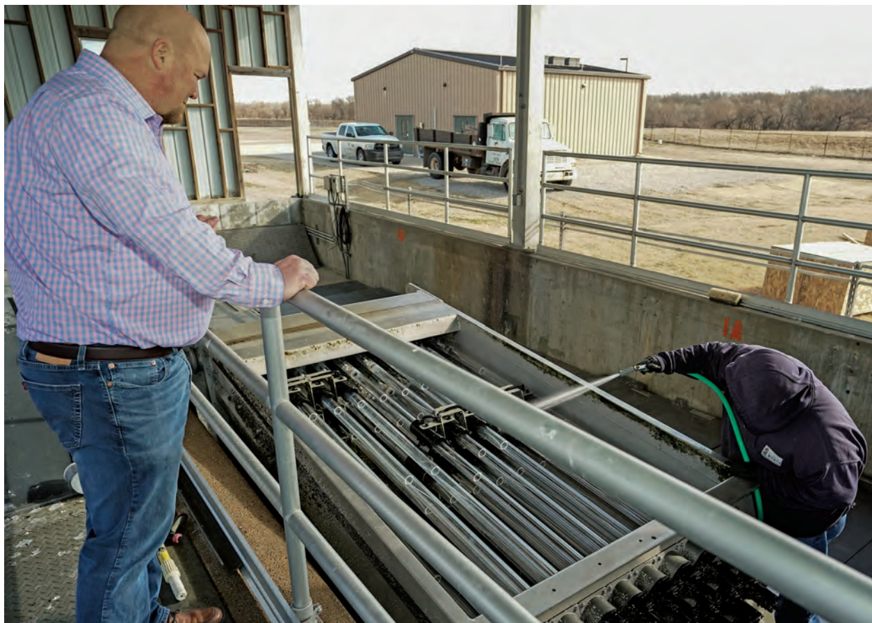
Jamie Belden, operations supervisor, watches worker Vicente Hernandez clean the lamps in the UV disinfection system (Trojan Technologies) installed at the Lower Arkansas River Wastewater Treatment Facility.
