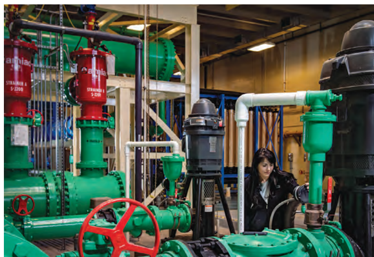
Kristen Reaves takes a reading of pump discharge gases (water filtration system from Amiad).
