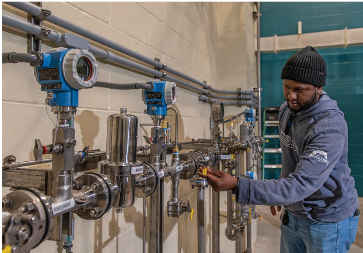
Operator Alpha Camara checks the valves in the ozone production room (Primozone).
