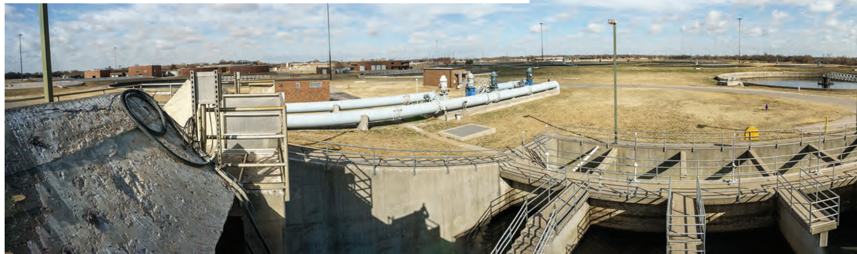
A general view of the Parkson OxyCharger static aerators installed at the Lower Arkansas River Wastewater Treatment Facility.
