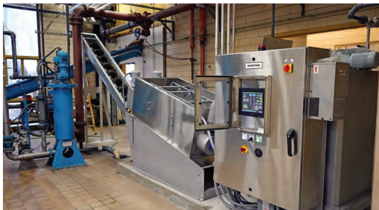
The unit's 149-by-52-inch footprint enabled installation next to the previous press.
