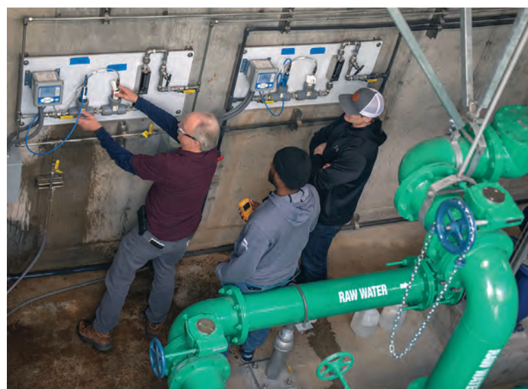
From left, Andrew Dieter, Alpha Camara and Mitchell Horner in the raw water vault, cleaning the ozone analyzers (Emerson/Rosemount).
