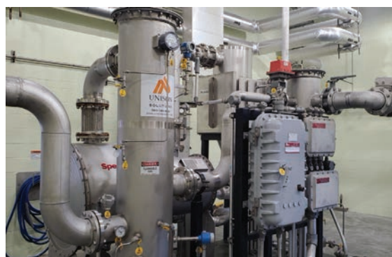
Unison Gas Compressors used to supply biogas to boilers.
