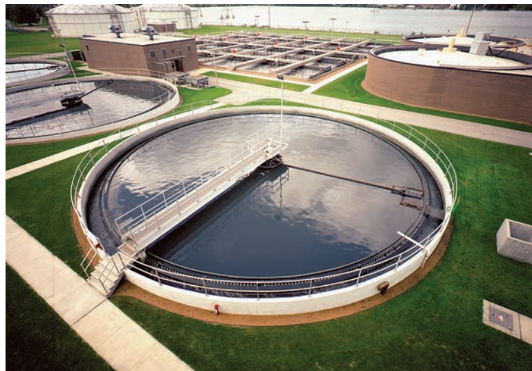
Between corrosion, maintenance, and changes in flow, keeping a clarifier working at peak performance can be challenging. Complimentary inspection by OEMs for circular or rectangular clarifiers help assess equipment condition and performance. (Tow-Bro clarifier from Evoqua Water Technologies)
