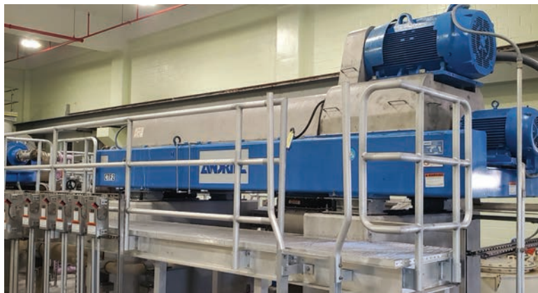
Andritz centrifuge in biosolids dewatering building.
