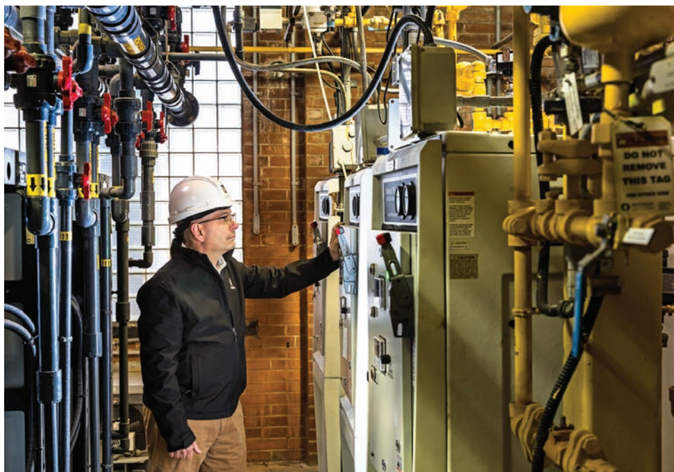
Locco is pictured at a bank of evaporators. A Wallace and Tiernan Series 50-200 evaporator (Evoqua Water Technologies) on the right side converts liquid chlorine to gas, which is sent to a bank of Wallace & Tiernan chlorinators and mixed with treated water.
