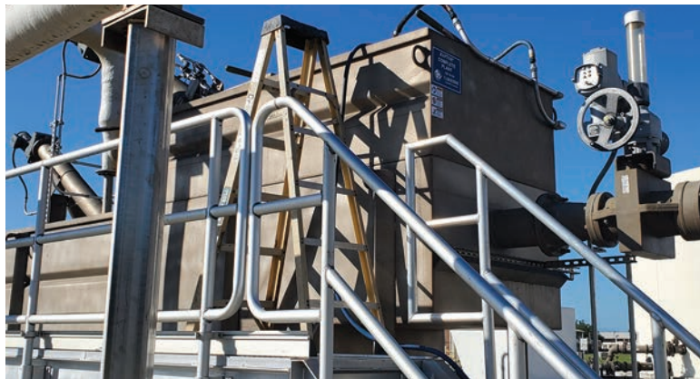
Lakeside Screening equipment located in the new septicage facility.
