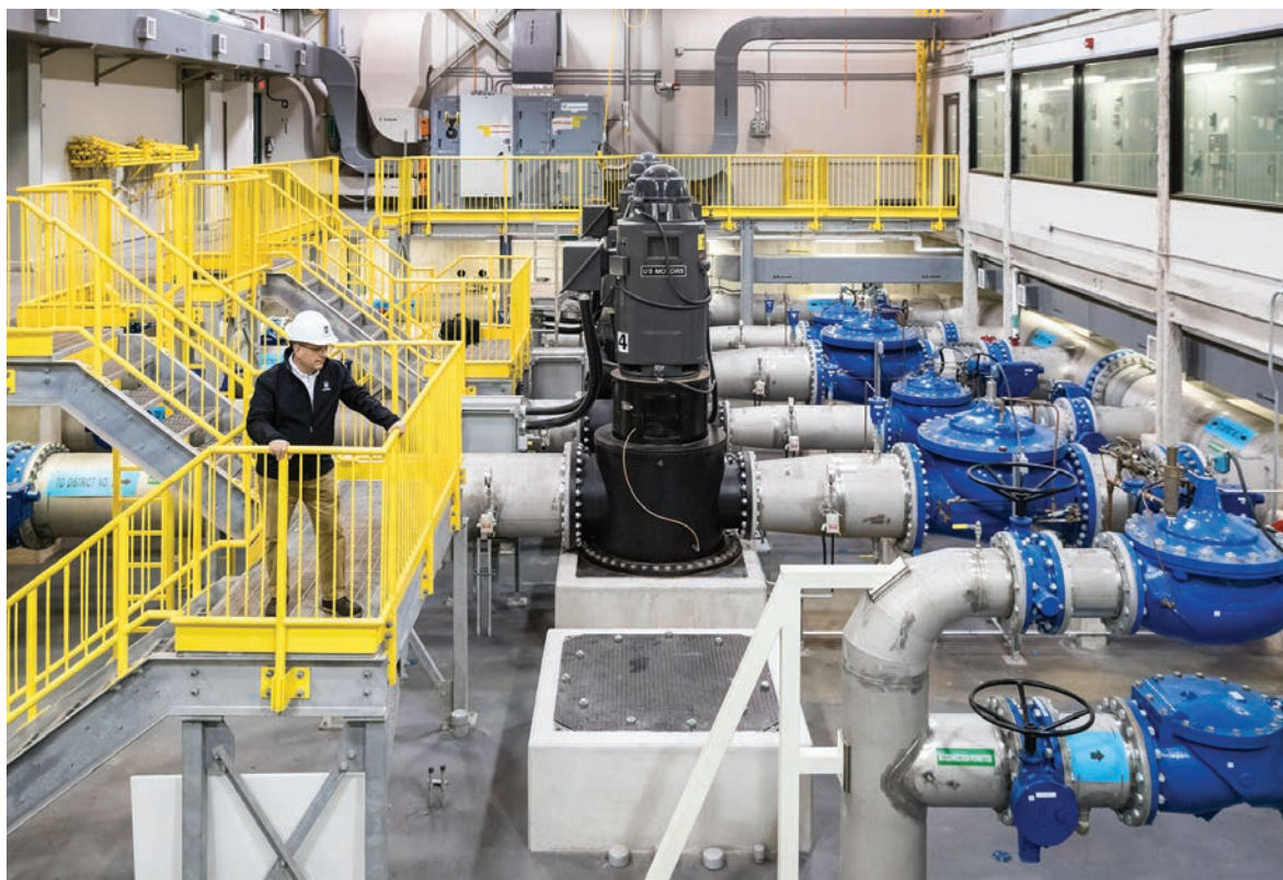
Locco in the Ferguson Pumping Station. The Goulds Vertical Industrial Can-Type pumps have US Motors (Nidec) motors; valves are Cla-Val.
