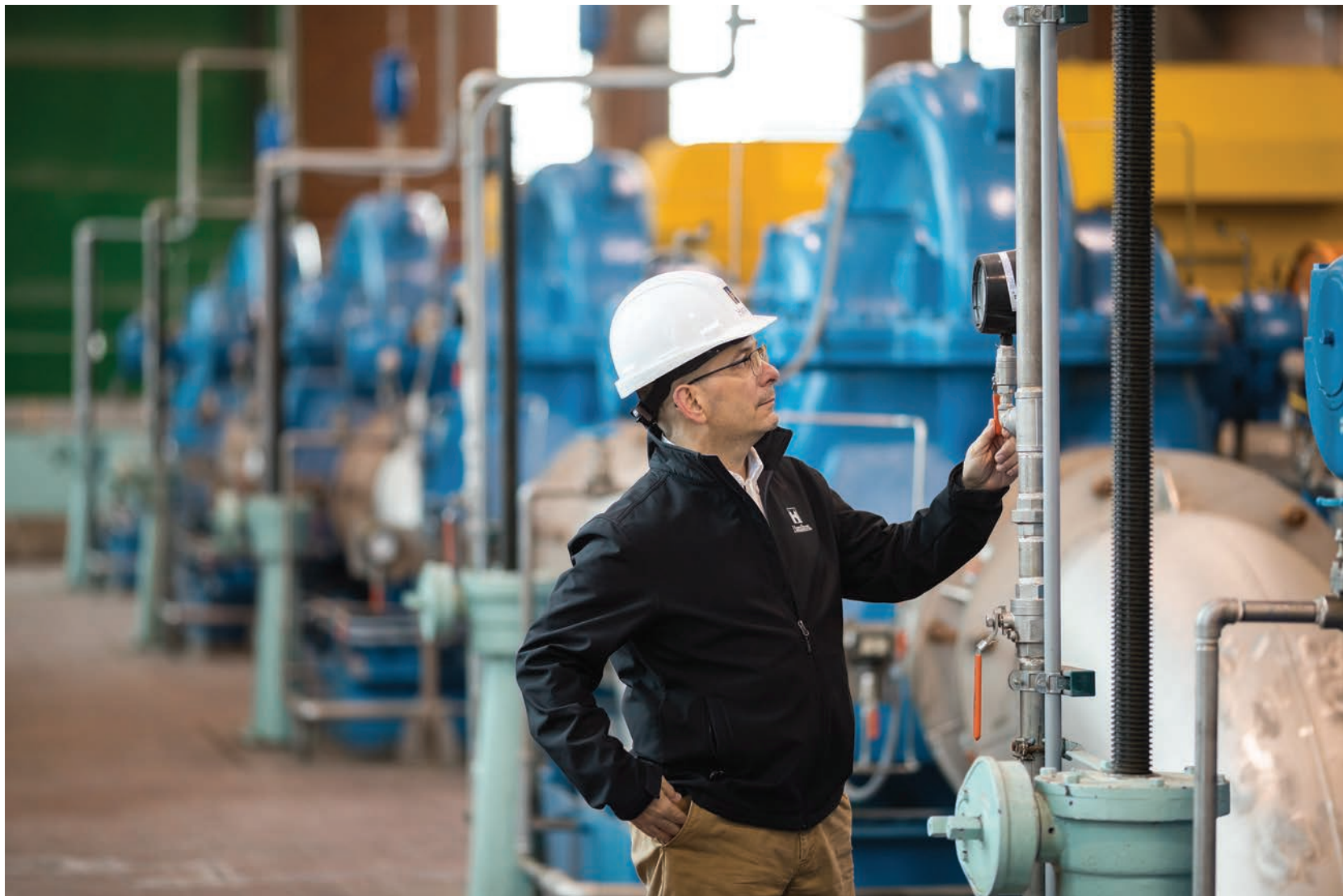
Danny Locco inside the Woodward Avenue Wastewater Treatment Facility pump station, with a bank of six high-lift Goulds pumps, Model 3498, with 24,000 gpm capacity, each powered by a 1,900 hp TECO-Westinghouse 4,160 V motor.
