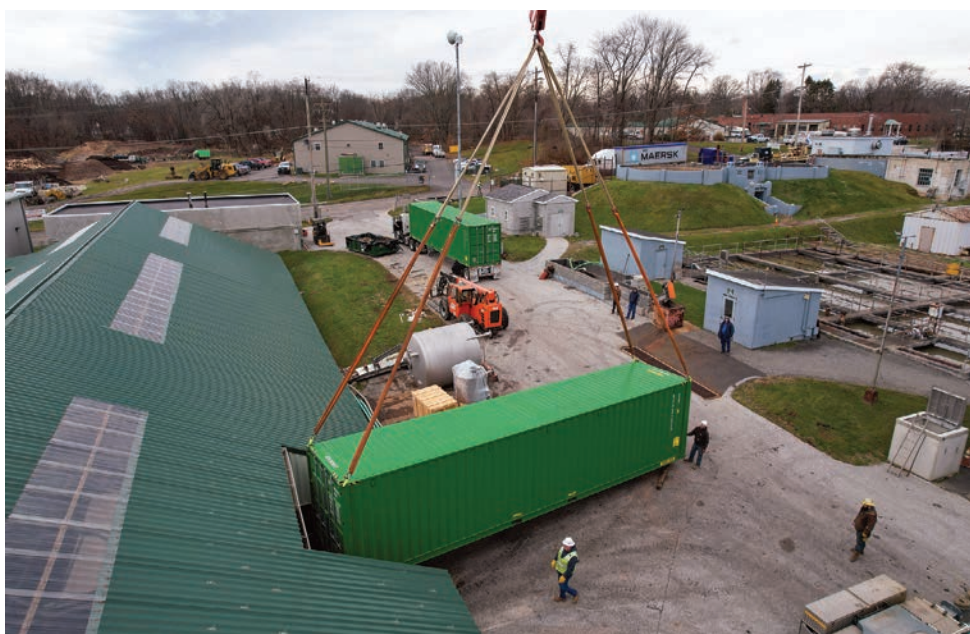
Shipping containers holding the reactor and the heat exchanger for hydrothermal carbonization were moved into a building at the Phoenixville treatment plant.
