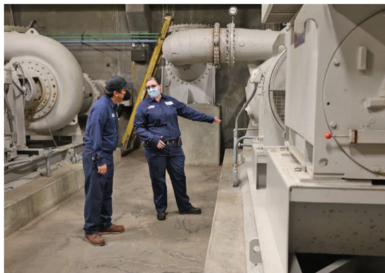
This TECO-Westinghouse three-phase induction motor powers 300 hp, 490 rpm interstage pumps with adjustable-speed magnetic drive clutch that send water from the primary sedimentation structure effluent channel into the trickling filters.
