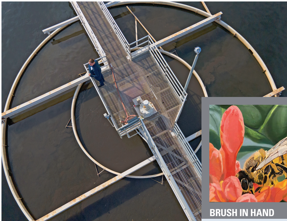
An aerial view of the secondary clarifiers at the Santa Cruz plant (clarifier drives by WesTech Engineering).
