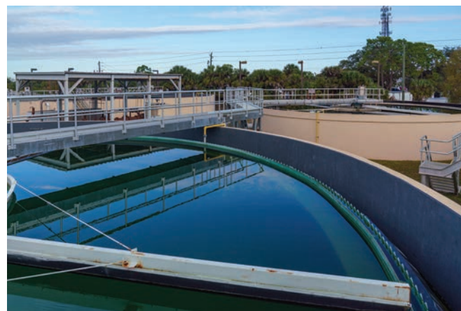
Four circular clarifiers precede four deep-bed sand filters.
