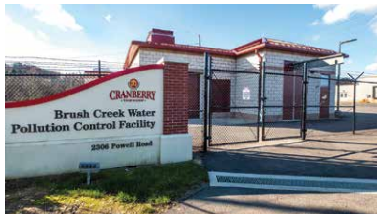
The Brush Creek Water Pollution Control Facility has a design flow of 6 mgd and treats an average of 3.4 mgd. It uses a membrane bioreactor process.
