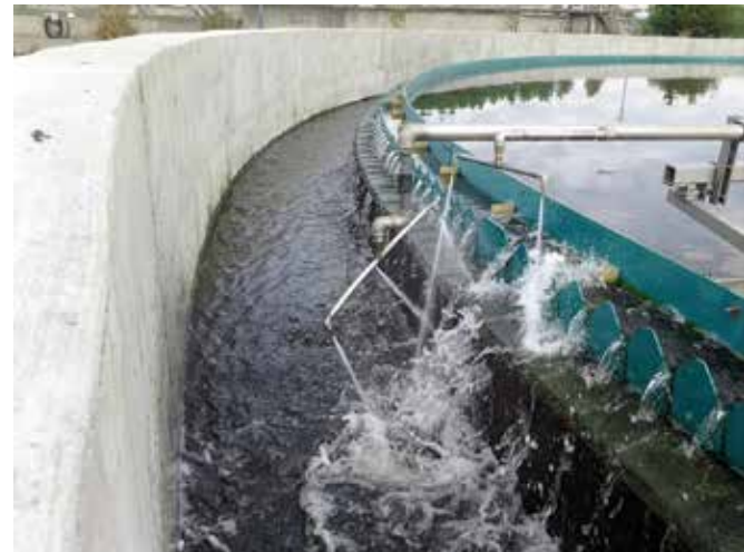
Automated weir washers remove algae, grease, sludge and other materials from the weirs, baffles and launders in clarifiers, thickeners and other tanks.
