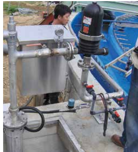
To break up and remove algae from wastewater tanks, two workers are typically required, often for several hours per day.
