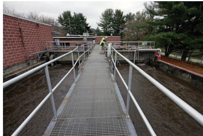
The Richmond treatment plant has a dry-weather design capacity of 222,000 gpd and treats an average of 70,000 gpd.
