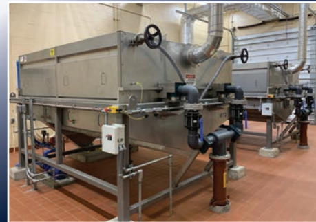
Dual 4 x 10 Rotary Drum Thickener
