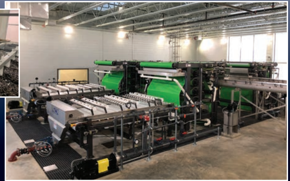
Independent Gravity Zone of 3DP Belt Press
