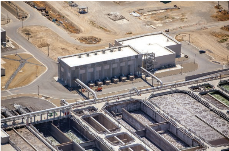
The Sacramento plant operated by Regional San is the largest discharger to an inland water body west of the Mississippi River. It treats 130 mgd on average and has capacity to treat up to 330 mgd.
