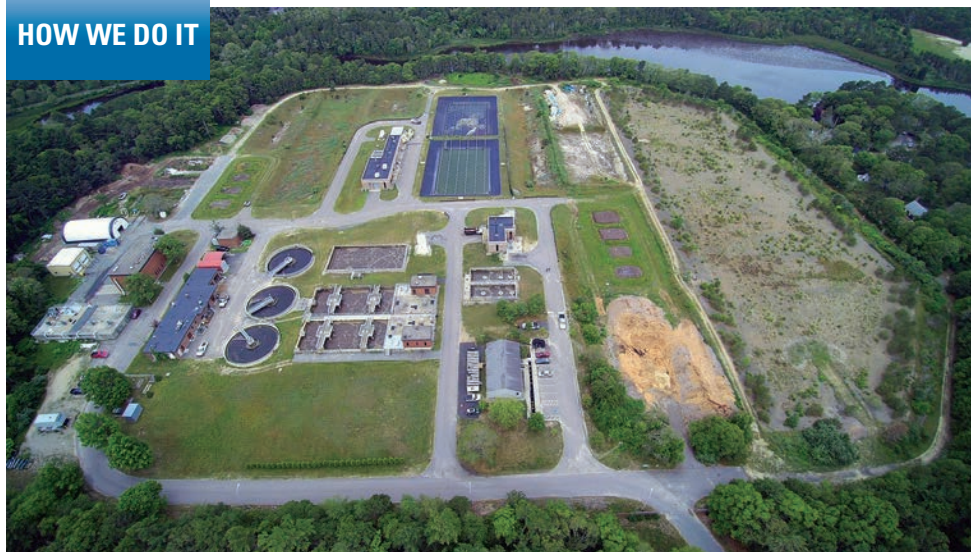
The Wareham Water Pollution Control Facility is fed by 61 miles of gravity sewer pipe and 45 pump stations. It treats 1.56 mgd with biological nutrient removal.
