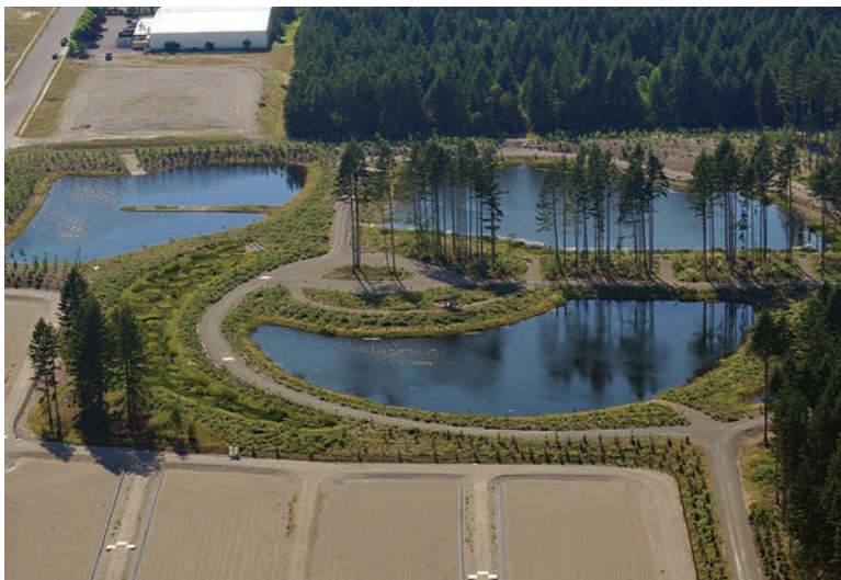
Hawks Prairie Ponds is one site where the LOTT Clean Water Alliance recharges the aquifer with Class A reclaimed water.
