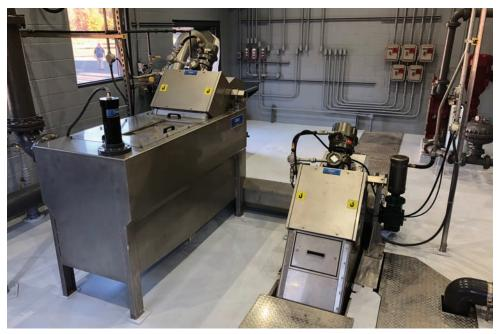
A 6 mm step screen and 2 mm step screen-in-tank (both from Claro Environmental Technologies) protect an MBR system as well as a common wash press unit complete with bagger.
